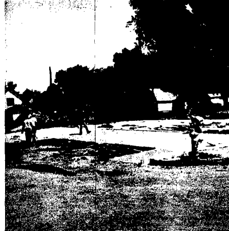
FIREHALL CONSTRUCTION at Carroll is underway. Crewmen from Gerhold Concrete Co., Norfolk, were finishing up the concrete floor Thursday. The new building will feature four stalls and four doors for four vehicles. Measuring approximately 40 by 80 feet, the building will be made of steel. Front of the building will open to the west, facing mainstreet Carroll's city park edging the lots on the south. Quarters for firemen's meetings will be located in the west end of the structure.
